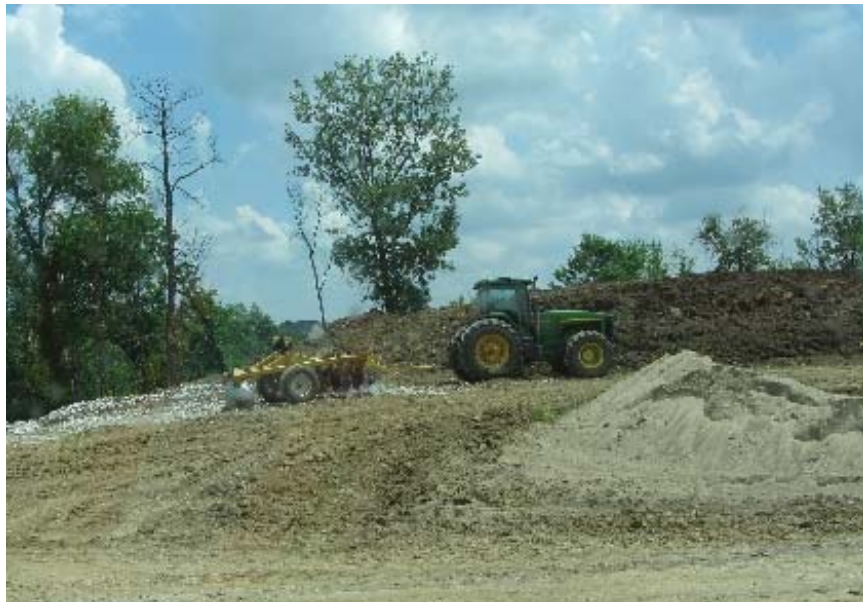
Figure 31. Disk used to dry embankment materials
