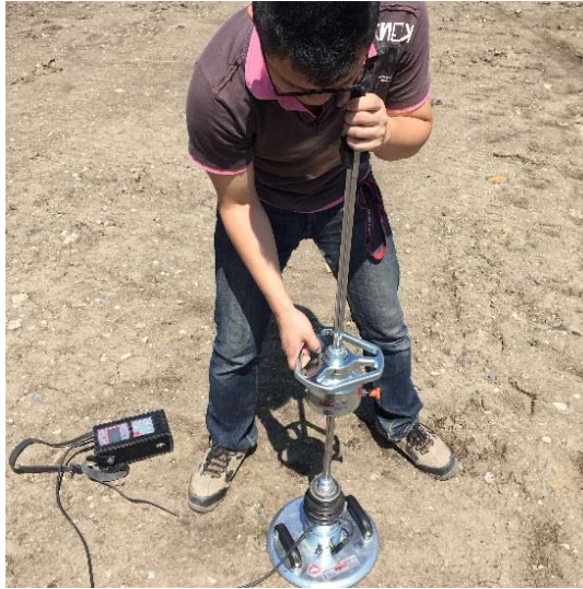
Figure 10. Light weight deflectometer test
