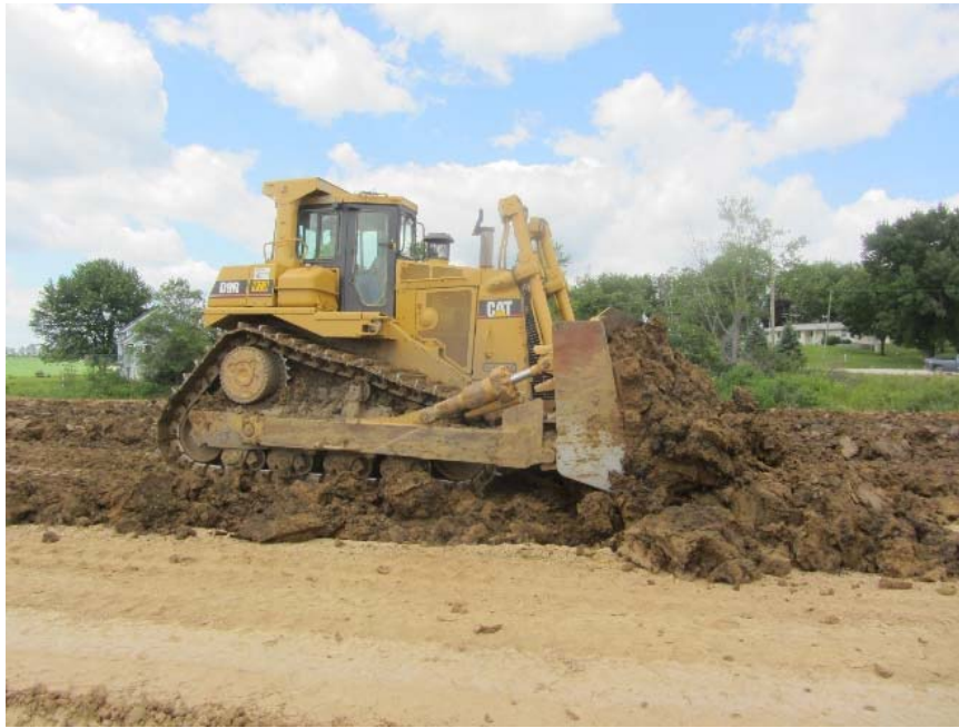
Figure 54. Caterpillar D6R Dozer used to control lift thickness
