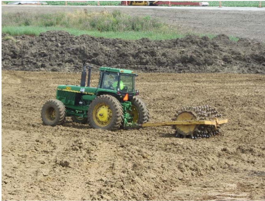
Figure 79. Sheepfoot roller used for soil compaction
