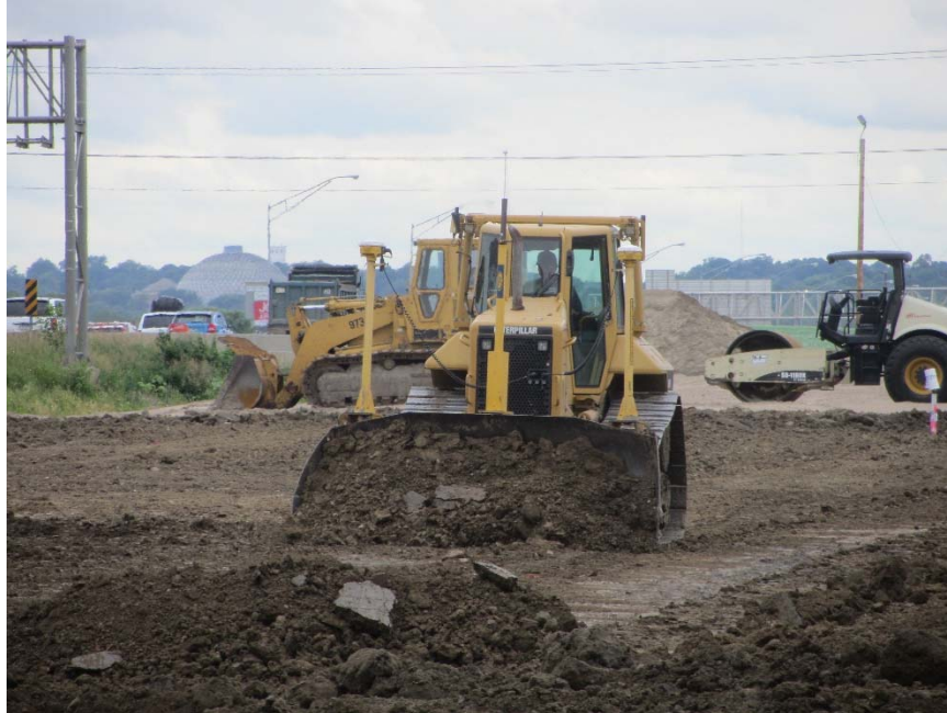
Figure 86. Caterpillar dozer used to control lift thickness
