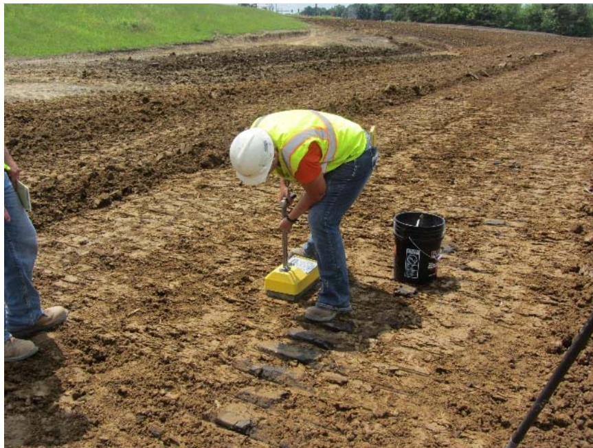
Figure 71. Contractor was conducting QC tests
