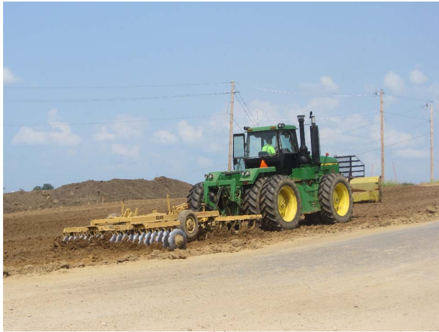
Figure 109. Disk used to dry embankment materials
