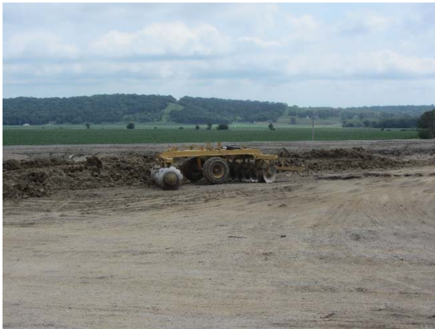
Figure 78. Disk presented on site without pulling machine
