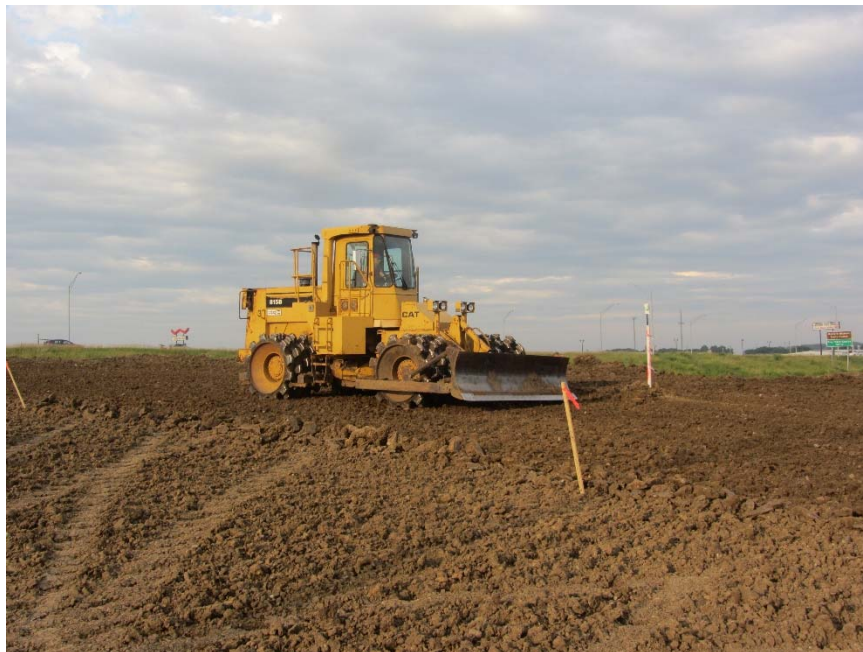
Figure 87. Caterpillar 851B dozer with sheepfoot roller wheel used for soil compaction
