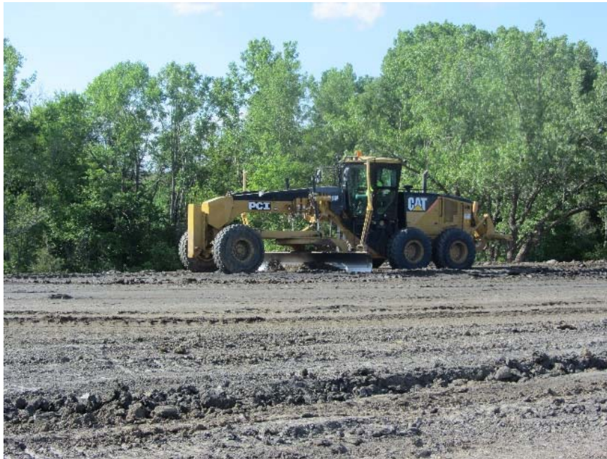
Figure 57. Caterpillar 14M motor grader used to level the embankment surface
