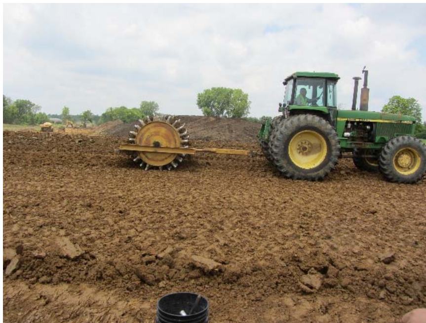
Figure 69. Sheepfoot roller used for soil compaction
