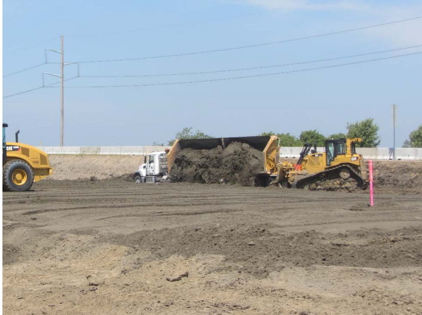
Figure 95. Dump truck used to place loose fill materials
