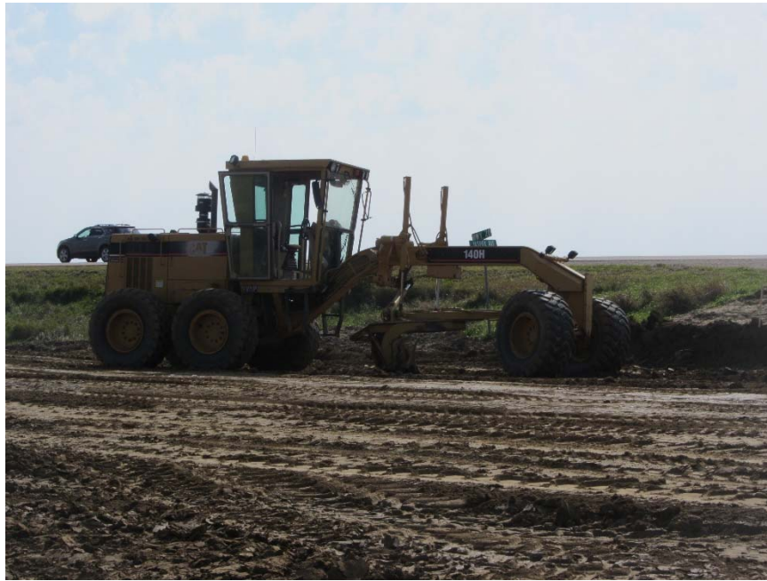
Figure 121. Caterpillar 140H motor grader used to level the embankment surface
