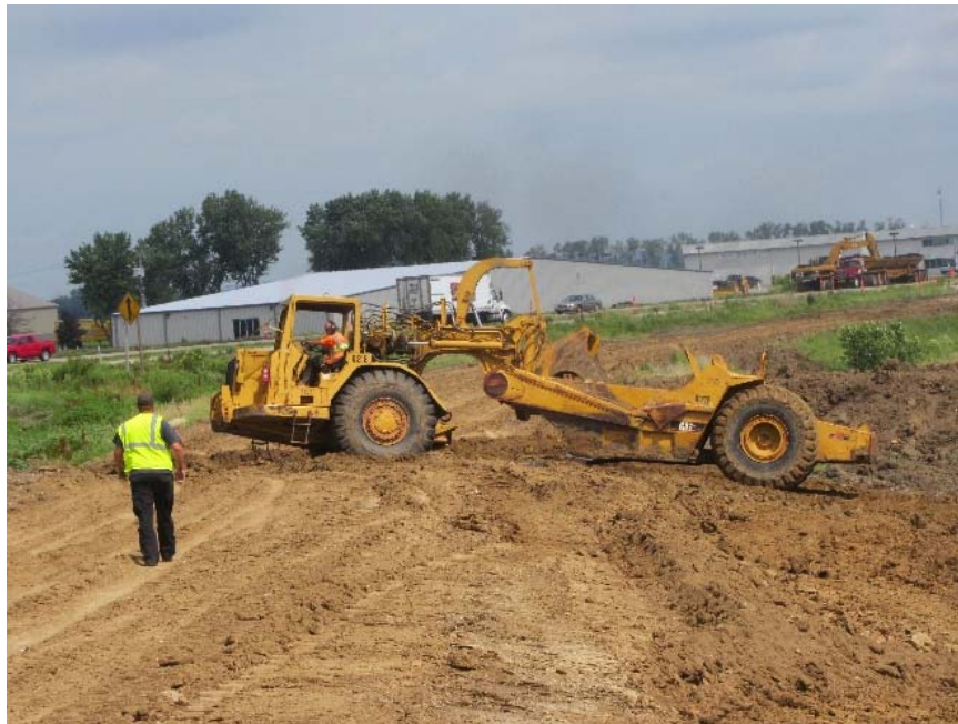
Figure 76. Caterpillar 621E scraper used to collect and place loose fill materials
