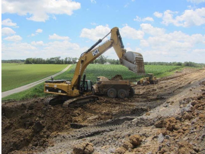
Figure 53. Caterpillar 390D excavated materials from borrow source
