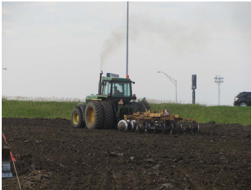
Figure 89. Disk used to dry embankment materials
