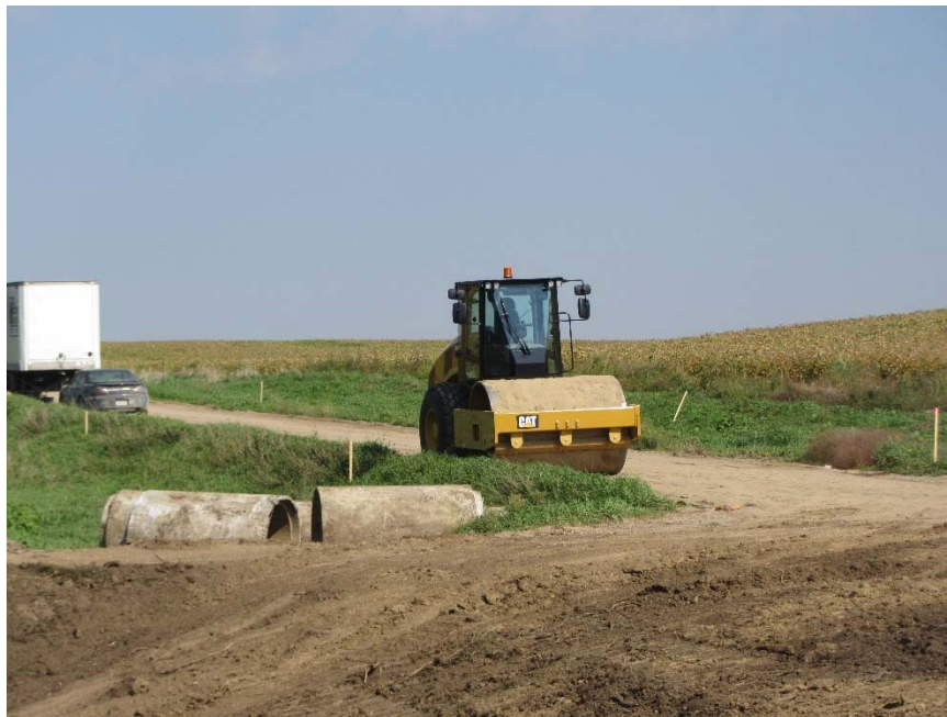
Figure 122. Caterpillar CS56 series vibratory smooth drum roller used for soil compaction
