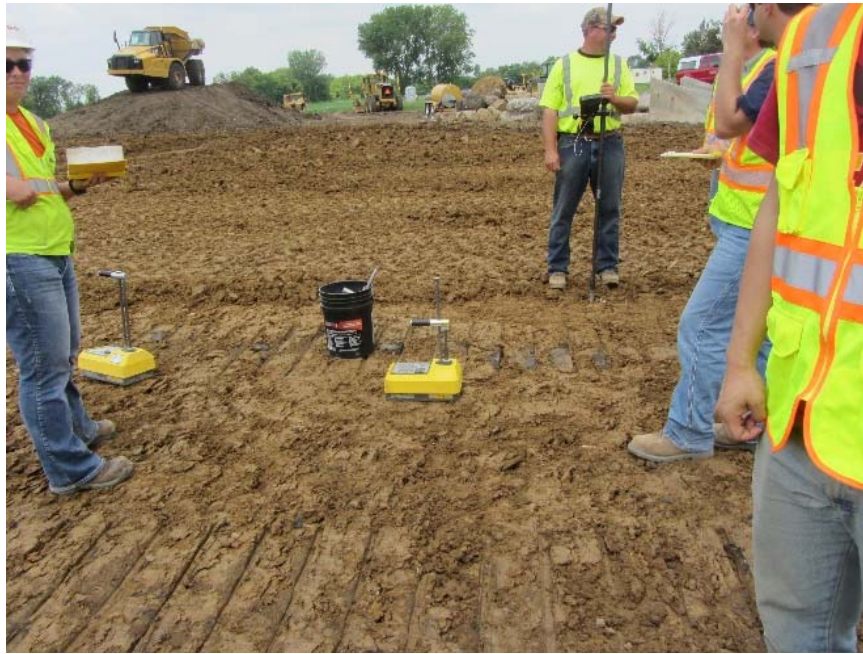
Figure 72. DOT engineer was conducting QA tests
